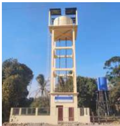
Figure 2: RWC Community piped water supply system in Dang Kambet commune
