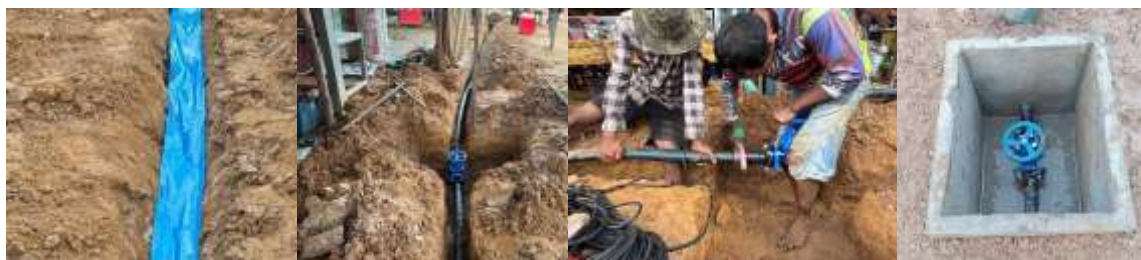
Figure 3: Water supply system and inauguration ceremony in Dang Kambet commune, featuring 80 meters borehole, an 18 meters water tower, 4000 pipe network and solar/gravity reticulation up to 200 households, all managed by an elected commune management committee.
